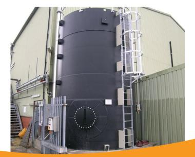
Salt is delivered via the delivery line and is directed to sit on the top of the 2-layer gravel bed. Water is introduced and percolates through the salt, with the water dissolving the salt layer as it passes through.
